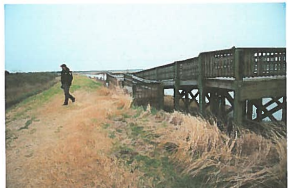
Observation deck on lake; to be connected with a trail spur
