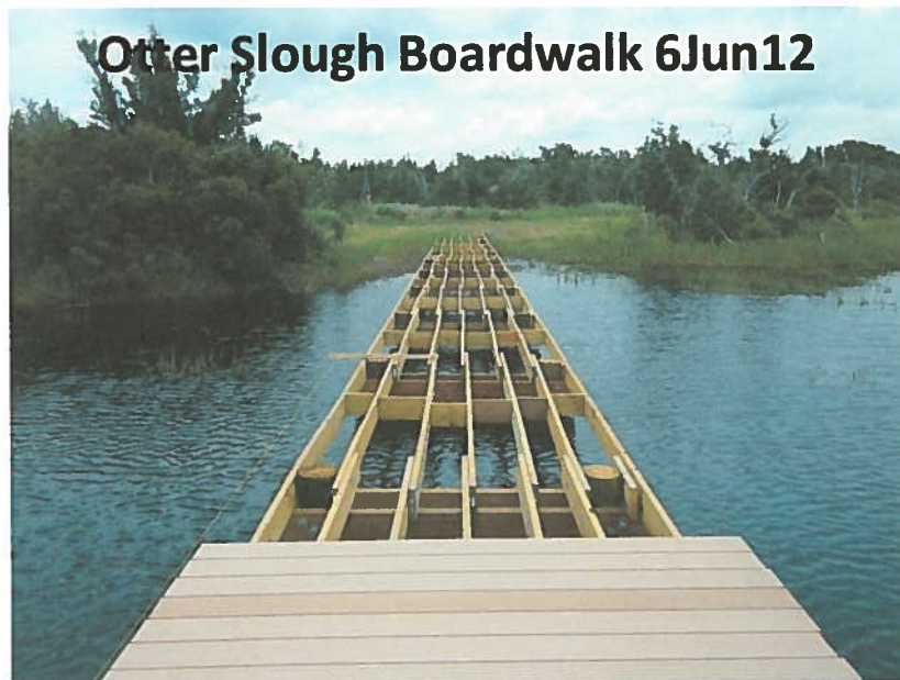
Example of boardwalk construction methods over water.
